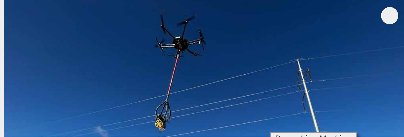
Drone Line Marking
