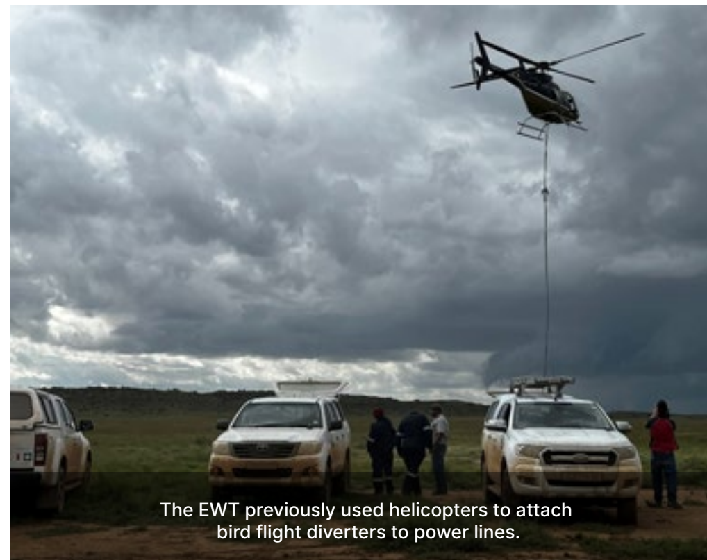
The EWT using a helicopter to attach bird flight diverters to power lines.
