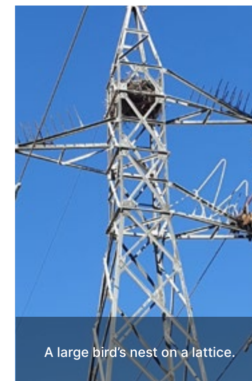
A platform installed on a distribution tower for birds to nest on safely, reducing mortalities and preventing damage to the infrastructure.
