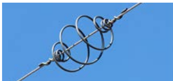
Bird-friendly structure (left). Photo credit: Constant Hoogstad. Raptor guards fitted to a T-pole to prevent a potential electrocution on the pole top (top right). Photo credits: Power Line Sentry. Bird flight diverter fitted to a conductor on a transmission line to make the line more visible and reduce bird collisions (bottom right). Photo credit: Marianne Golding
