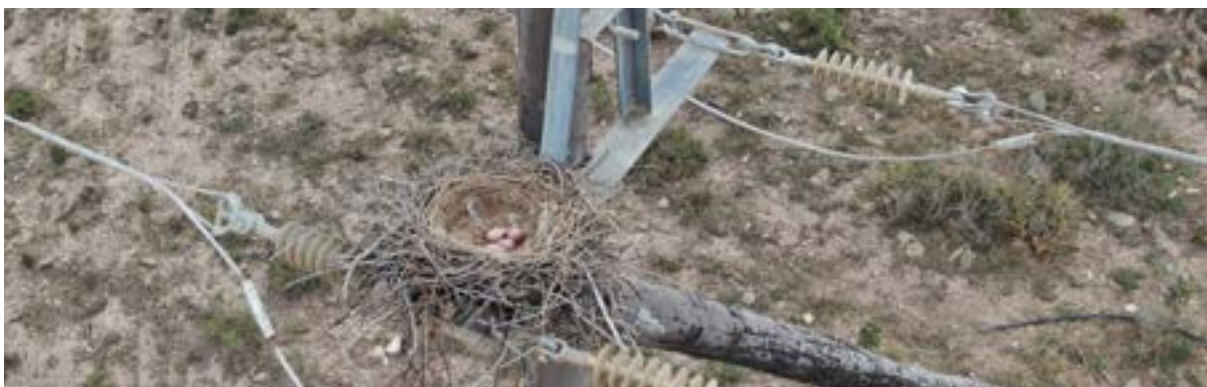
Red-billed Buffalo Weaver nesting on a structure close to critical hardware (top left) and on a nesting platform (top right). Photo credit: Werner Sieburg. Cape Crow nest on an A-frame strain structure (bottom). Photo credit: Matt Pretorius.
