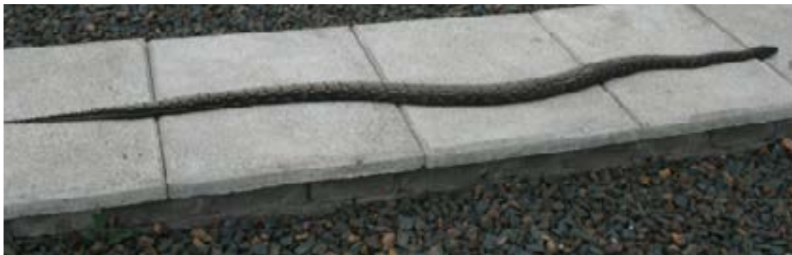
African Rock Python electrocuted in a substation. Photo credit: Eskom
