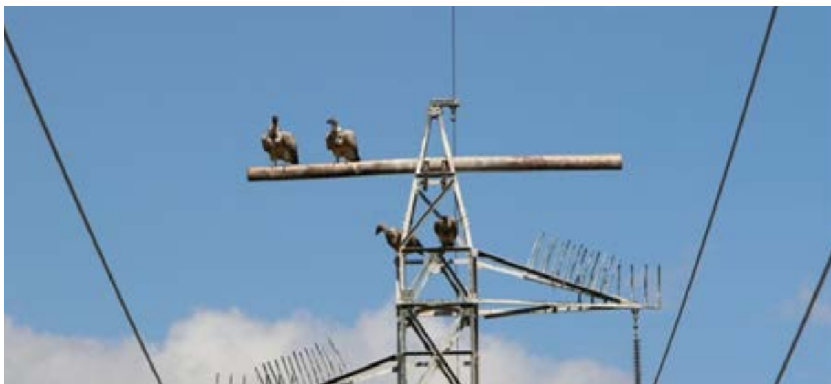
Cape Vultures roosting on a distribution structure. Note the 'white wash' on the structure from birds defecating. Photo credit: Constant Hoogstad
