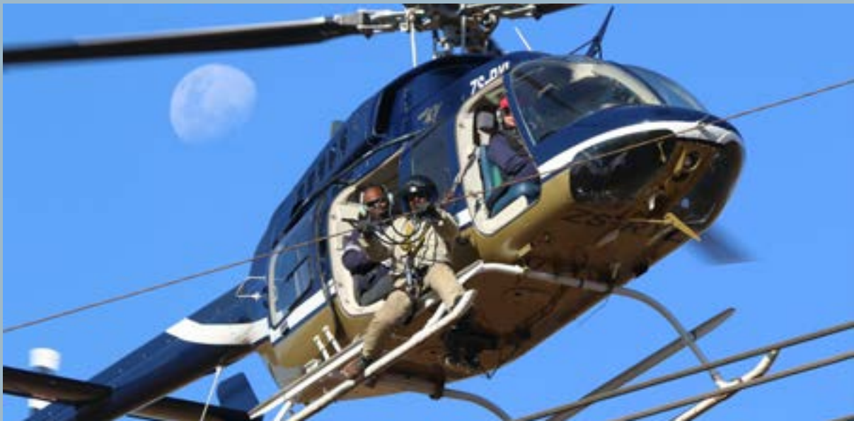
Installation of bird flight diverters from a helicopter by live-line personnel. Photo credit: Constant Hoogstad
