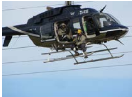
The Rotamarka device installed at Vissershok landfill site (top). The Eskom live-line team installing Rotamarka devices by helicopter (bottom). Photo credits: Lourens Leeuwner (top and bottom)
