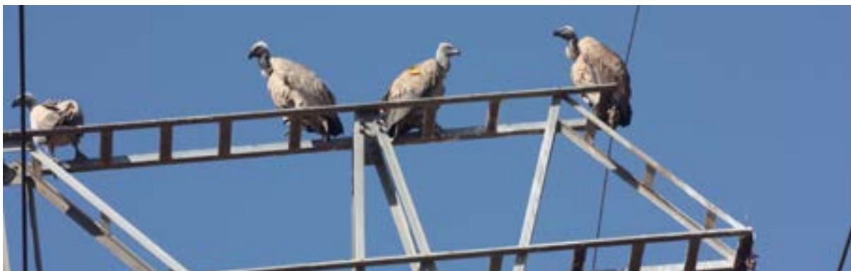
A White Stork electrocuted on a distribution power pole (top left). Photo credit: Ronelle Visagie A Brown Snake Eagle nest on a power line pole (top right). Photo credit: Andre Botha Cape Vultures roosting on a distribution tower (bottom). Photo credit: Constant Hoogstad
