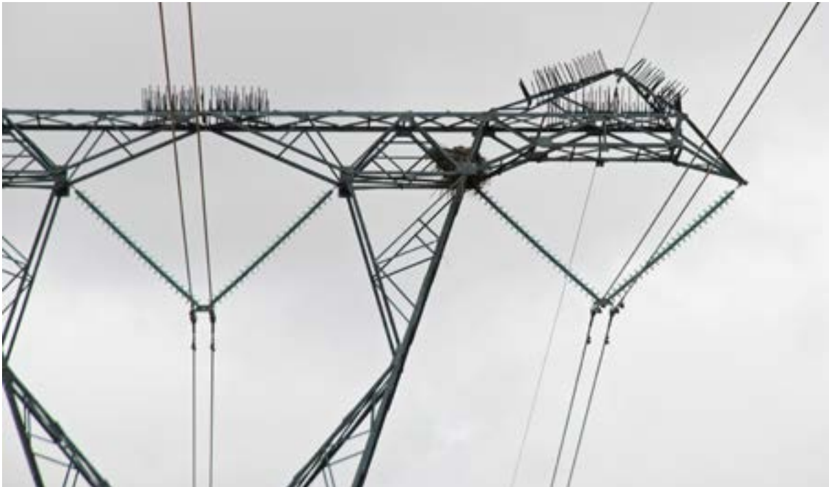
Verraux's Eagle nest located in a high risk area above an insulator on a transmission line.
