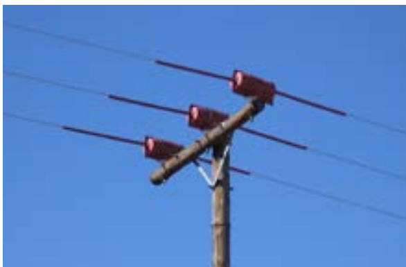
Raptor protectors fitted to a distribution pole top where bird electrocutions occurred (top left). Photo credit: the EWT. Raychem insulation products fitted to distribution pole top to reduce the amount of bird electrocutions. (bottom left). Photo credit: the EWT. An RPAS in flight attaching bird flight diverters to a live power line. (right). Photo credit: Eskom
