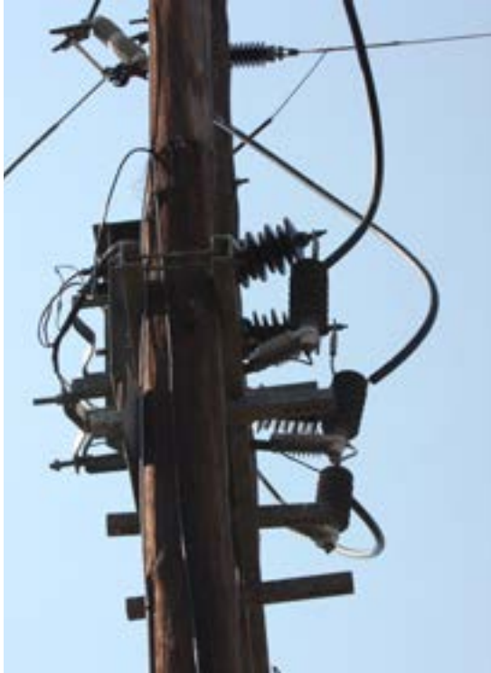
Transformer box (left) with exposed jumpers where Ground Hornbill was electrocuted (right). Photo credit: Constant Hoogstad (left) and Lucy Kemp and Mabula Ground Hornbill project (right)
