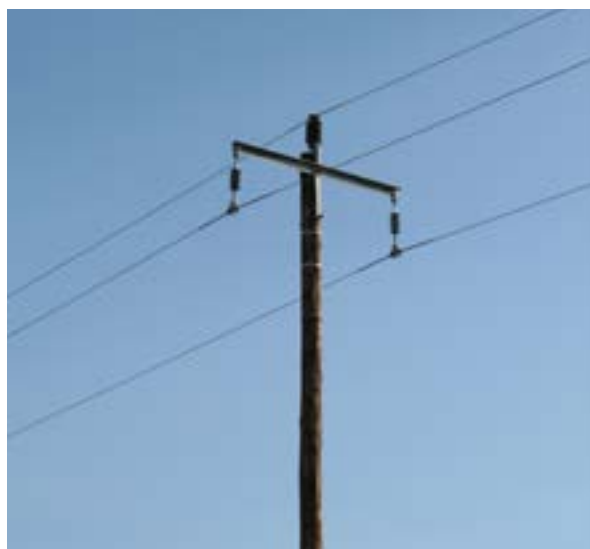
Bird-friendly structure (left). Photo credit: Constant Hoogstad. Raptor guards fitted to a T-pole to prevent a potential electrocution on the pole top (top right). Photo credits: Power Line Sentry. Bird flight diverter fitted to a conductor on a transmission line to make the line more visible and reduce bird collisions (bottom right). Photo credit: Marianne Golding
