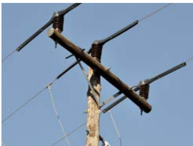
Wire bird guards (left) and raptor guards (right). Photo credits: Constant Hoogstad
