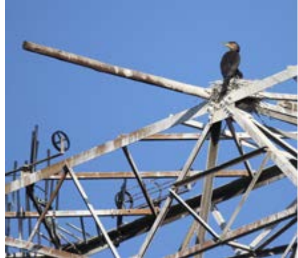
Reed Cormorants that are nesting, roosting, and polluting insulators on a transmission power line. Photo credits: Matt Pretorius
