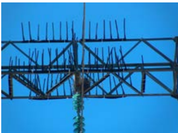
Perch guards fitted above the insulators on a transmission line to reduce the amount of streamer and pollution faults (top left). Photo credit: the EWT. Pied Crows nest built between perch guards fitted on a transmission tower (bottom left). Photo credit: Constant Hoogstad. Ground Hornbills perching on a structure above a transformer in Mabula game reserve, Limpopo Province, South Africa (right). Photo credit: Lucy Kemp / Mabula Ground Hornbill project.
