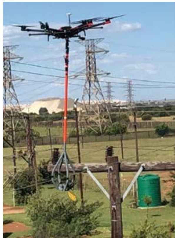
Raptor protectors fitted to a distribution pole top where bird electrocutions occurred (top left). Photo credit: the EWT. Raychem insulation products fitted to distribution pole top to reduce the amount of bird electrocutions. (bottom left). Photo credit: the EWT. An RPAS in flight attaching bird flight diverters to a live power line. (right). Photo credit: Eskom
