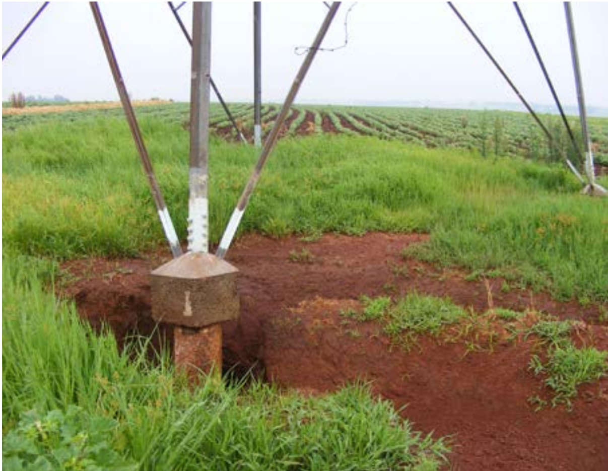
Porcupine burrows under transmission pylons in a maize field. Photo credit Constant Hoogstad
